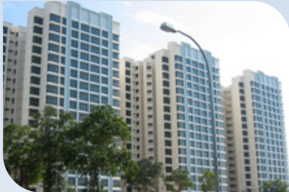
Apartments at Eunoss
