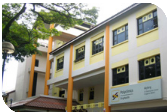
Polyclinic at Geylang East
